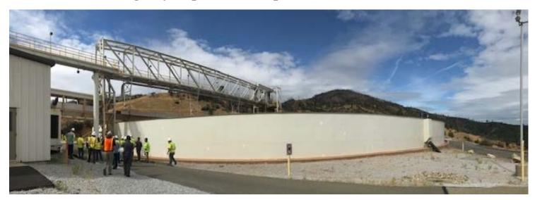
The afternoon tour of Iron Mountain Mine treatment plant was a rare opportunity for many of us to step foot on an active EPA Superfund Site. The acid mine drainage is treated with slaked lime (Calcium Hydroxide, Ca(OH)<sub>2</sub>) to neutralize the acid. The slurry is settled in a giant thickener tank (shown above). The red-colored sludge is dried in sludge drying beds before the sludge is transported to a disposal pit on site in one of the former mine's excavation areas.
